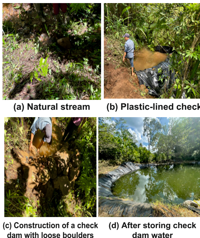
Fig. 53. (a-d) Flexible Check Dam for the Conservation of Water
